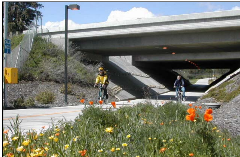
Putah Creek Bicycle Undercrossing
