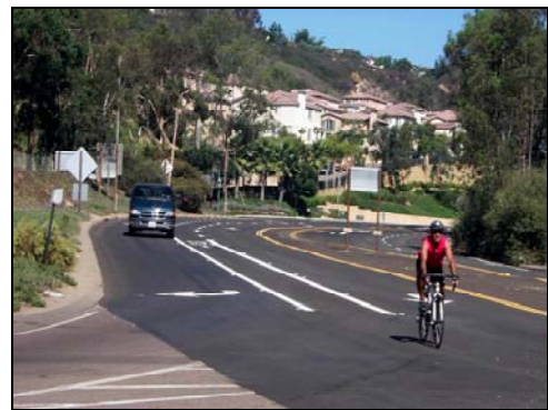
Gilman Drive at I-5 after being restriped and signed for improved bicycle access (San Diego)
