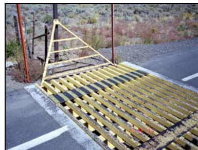
Innovative bike plates developed by Caltrans on S.R. 395 in Mono County help make cattle guards more bicycle-friendly.
