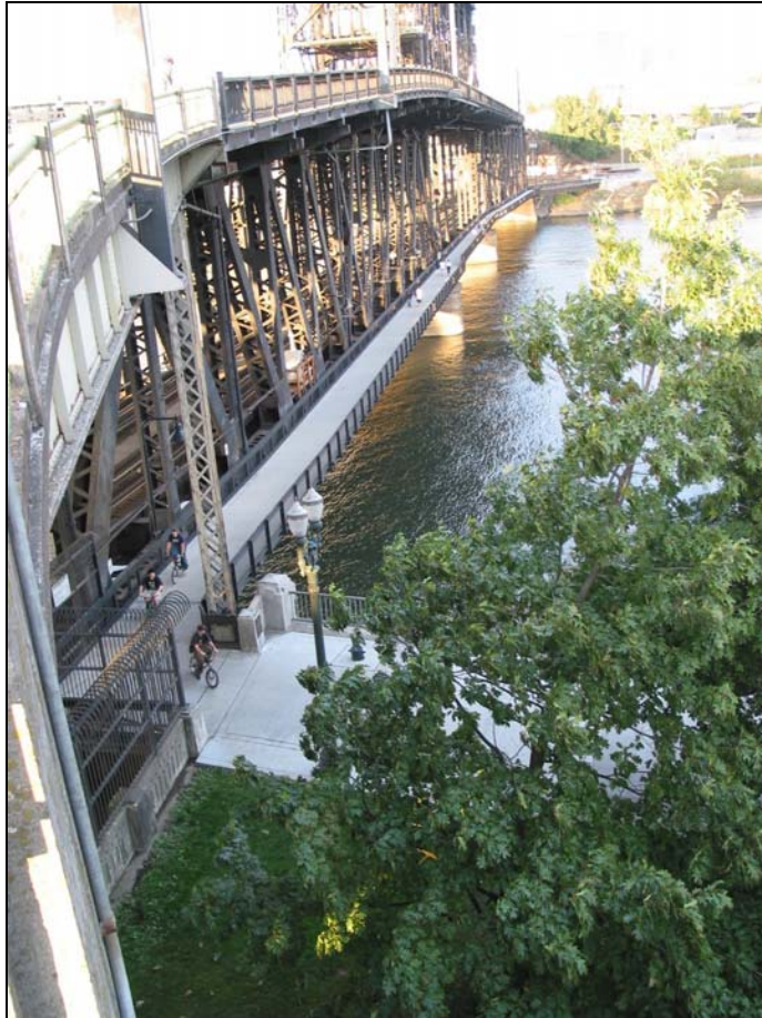
Steel Bridge RiverWalk, Eastbank Esplanade Portland, OR
