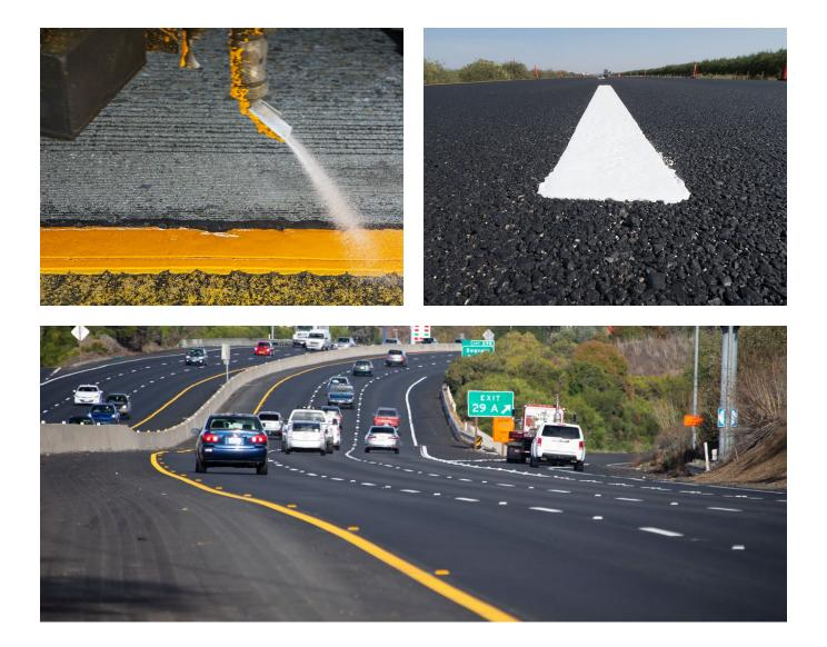
Caltrans has historically used 4-inch-wide painted stripes to delineate both edge and lane lines on the state highway system. More recently, Caltrans began deploying 6-inch-wide striping that uses more durable thermoplastic and tape.
