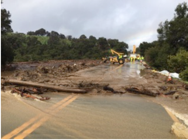
REPAIRS OVERTOPPING ROADWAY WITH TRACTORS ON SR 154 IN SANTA BARBARA COUNTY
