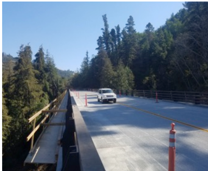
PFEIFFER CANYON BRIDGE OPENS AFTER REPAIRS, SR 1 IN MONTEREY COUNTY
