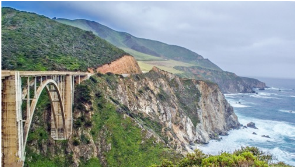
BIXBY CREEK BRIDGE ALONG SR 1 IN MONTEREY COUNTY
