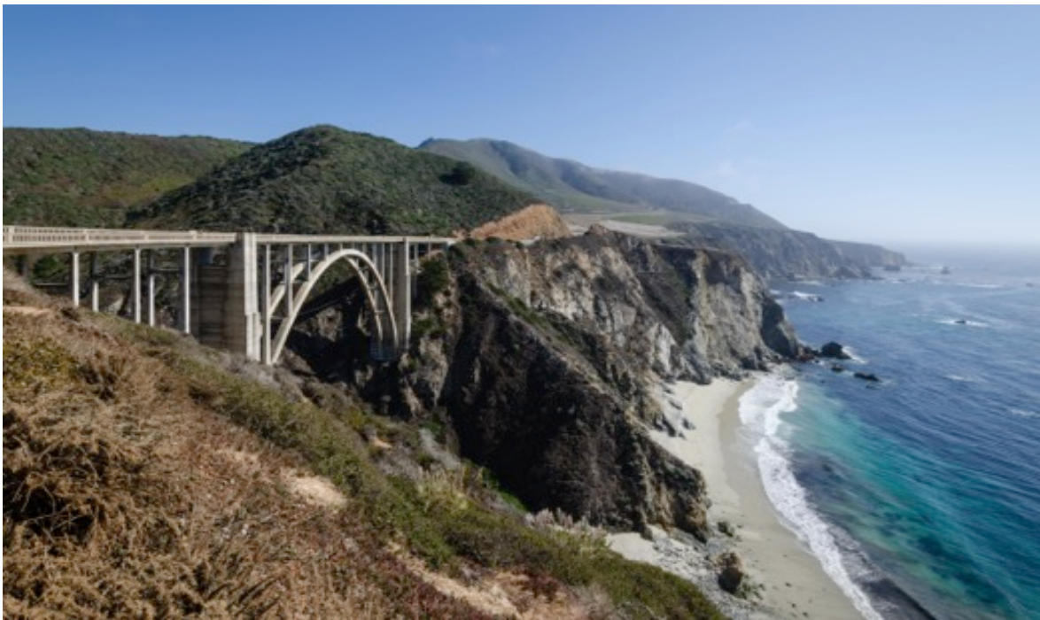
BIXBY CREEK BRIDGE, SR 1 IN MONTEREY COUNTY
