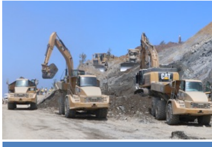
REPAIRS AND CLEAN UP AFTER MUDSLIDE ON SR 1 IN MONTEREY COUNTY
