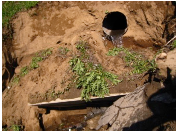
DRAINAGE FROM CULVERT ON I-10
