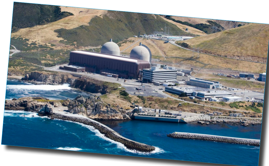
Diablo Canyon Nuclear Power Plant
