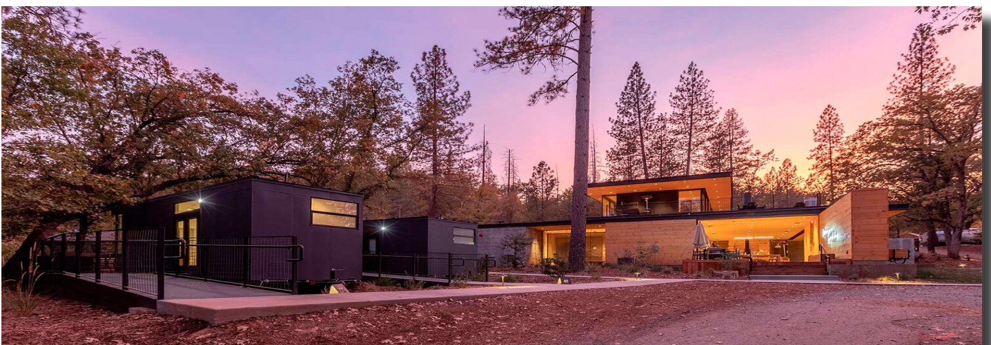
A rebuilt home that was destroyed by the Complex fire
