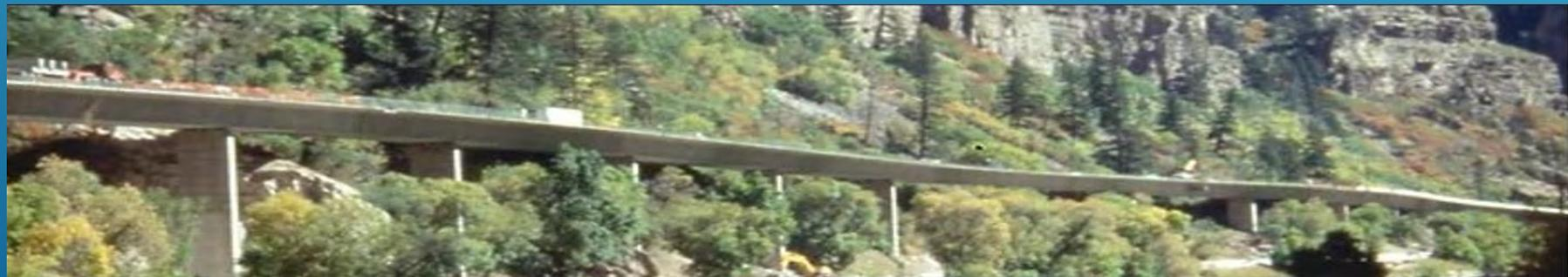
Viaduct example on I-70 in Colorado. Colored concrete matches local rock. Vegetation around viaduct columns visually integrates structure.
